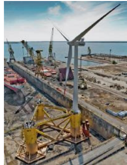
Figure: WindFloat in dry dock | source: Cermelli / Principle Power Inc.
