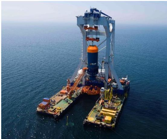
Fig. 1: The BLUE PILOT project aims at demonstrating a full scale monopile installation in the North Sea.
