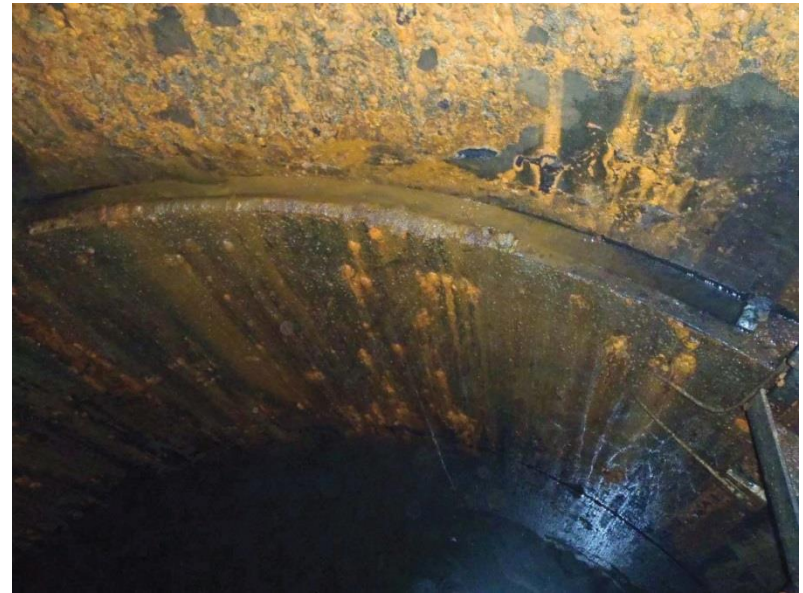
Insufficient inner corrosion protection
